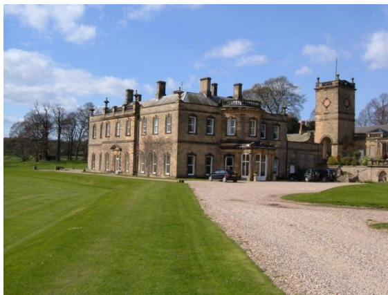
Hartforth Hall, Gilling, Yorkshire, purchased in about 1730 by William Cradock
