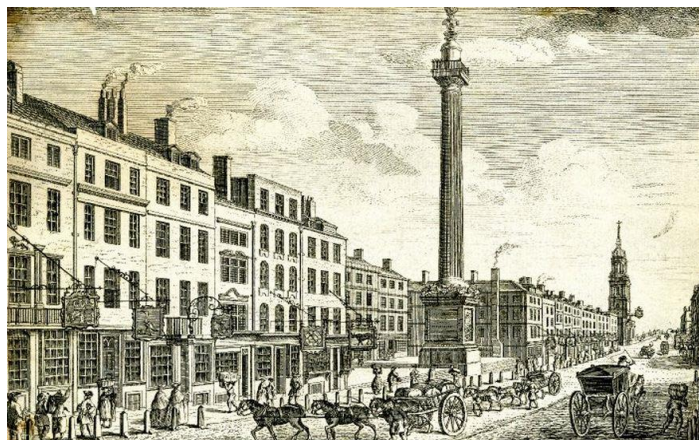
Above looking along Fish Street, toward the Monument and St. Magnus
