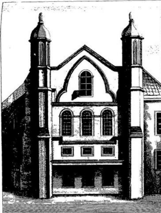
View of the HOUSE OF COMMONS from the River Thames.
