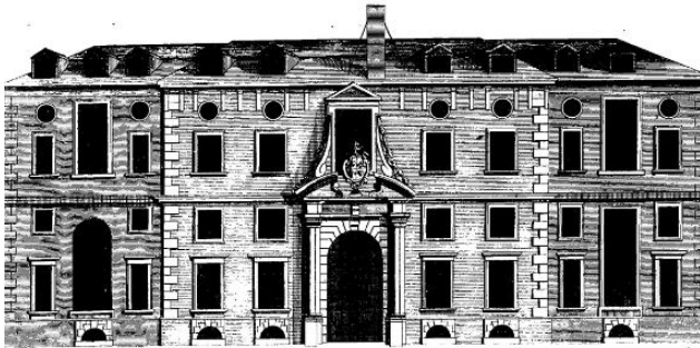
Goldsmith's Hall, in Foster Lane.
